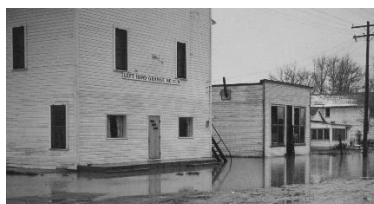
Street Flooding from Hinman Ditch
