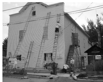
Restoration in Progress
